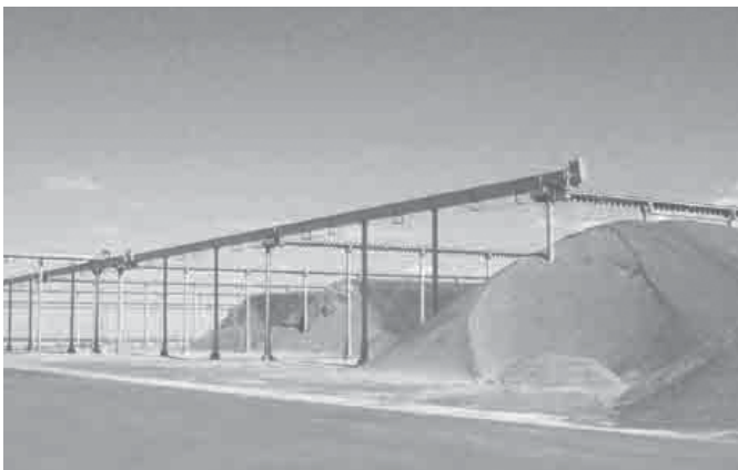
Partial view of a large outdoor installation employing leveling screws to spread material evenly across the storage area.
