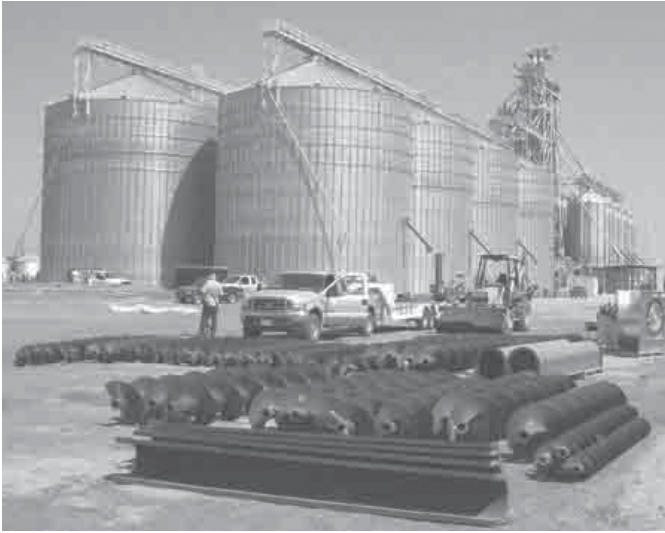
Typical installation of screw conveyors at a large grain storage facility.
